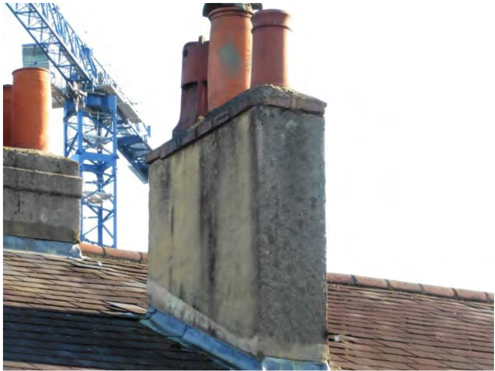
Rear stack viewed from the rear
