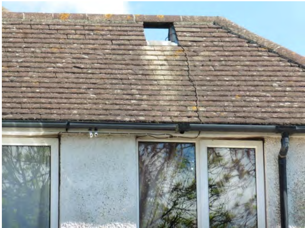
Rear roof pitch
