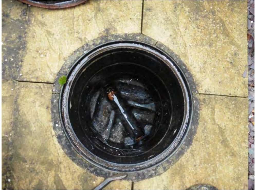
Inspection chamber to the front
