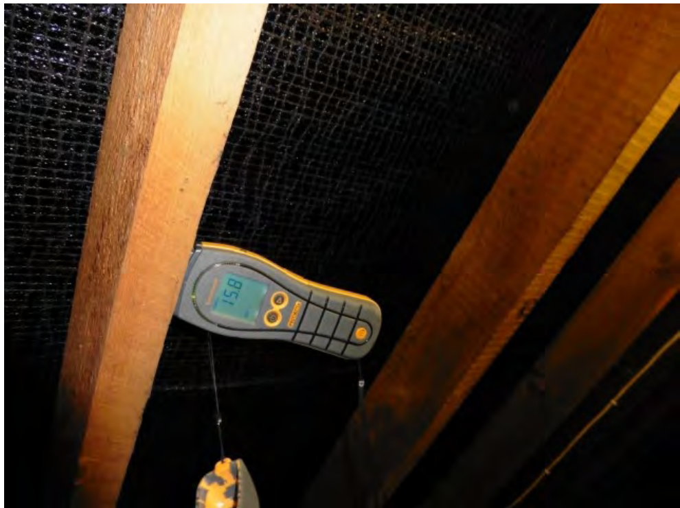
Normal moisture reading in roof timber
